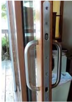
Mid 1990's Handle Only have Pins for a loose handle No parts for this.
