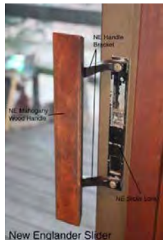
New Englander handle. Replacement parts generally available No locking mechanism Part # 620-3819 Approx. $15 each
